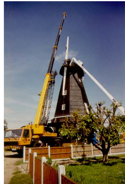
Fitting new laminated timber stocks
