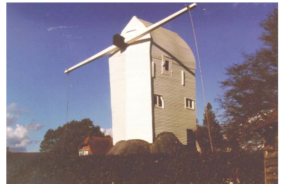
The mill on the 26 October 2002
