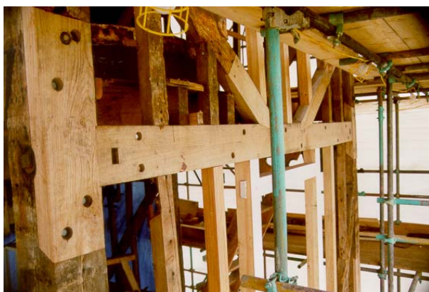
Major frame repairs
