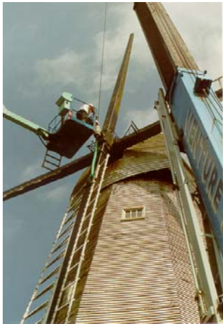
Removing the Dutch sails
