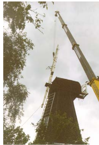
Removing the Steel Stocks
