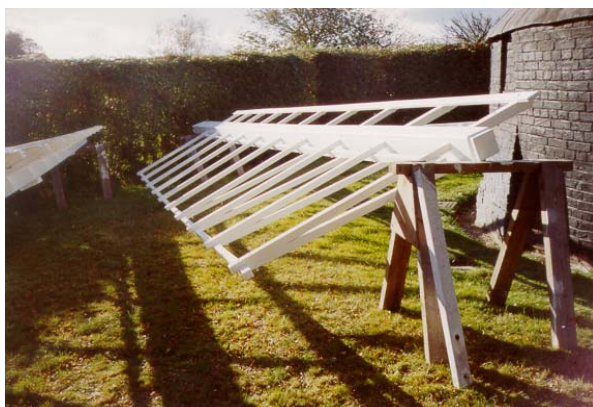
Sweeps removed for repair
