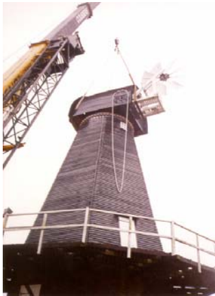
Replacing the Cap on 17 October 2002
