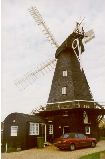
The work completed
