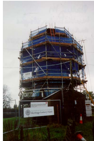
Weatherboarding stripped and frame repairs continuing 17 October 2002
