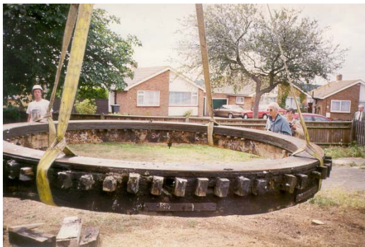
The old curb and cogs removed for rebuilding
